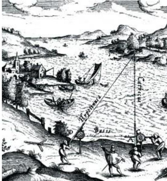
Measuring the width of a river by triangulation
